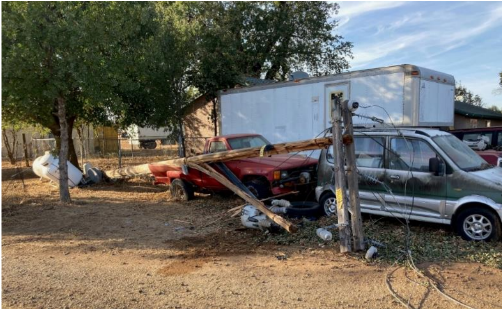
Figure 16: Wind damage in Shasta County – Broken Pole
