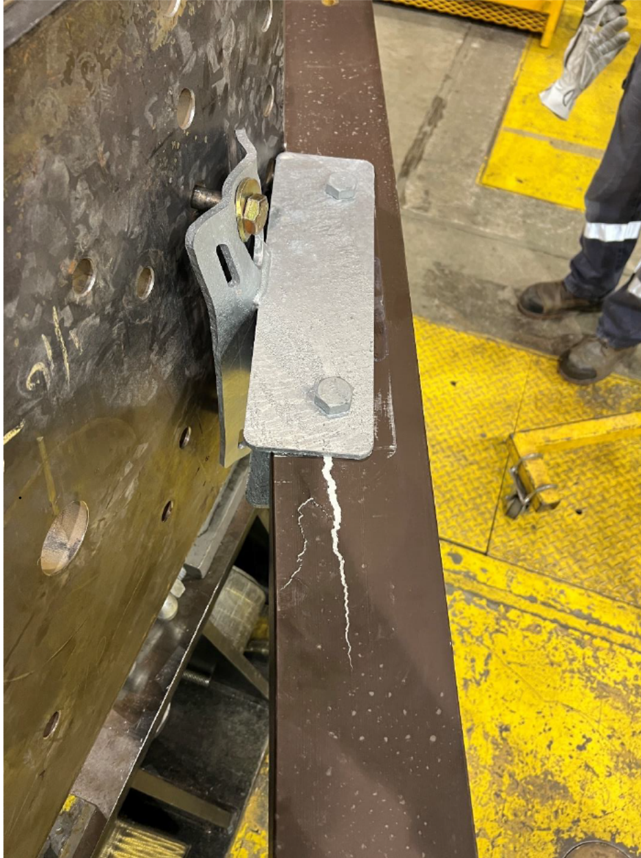
Figure 6-17: Sample 4.1 – Failure Location
