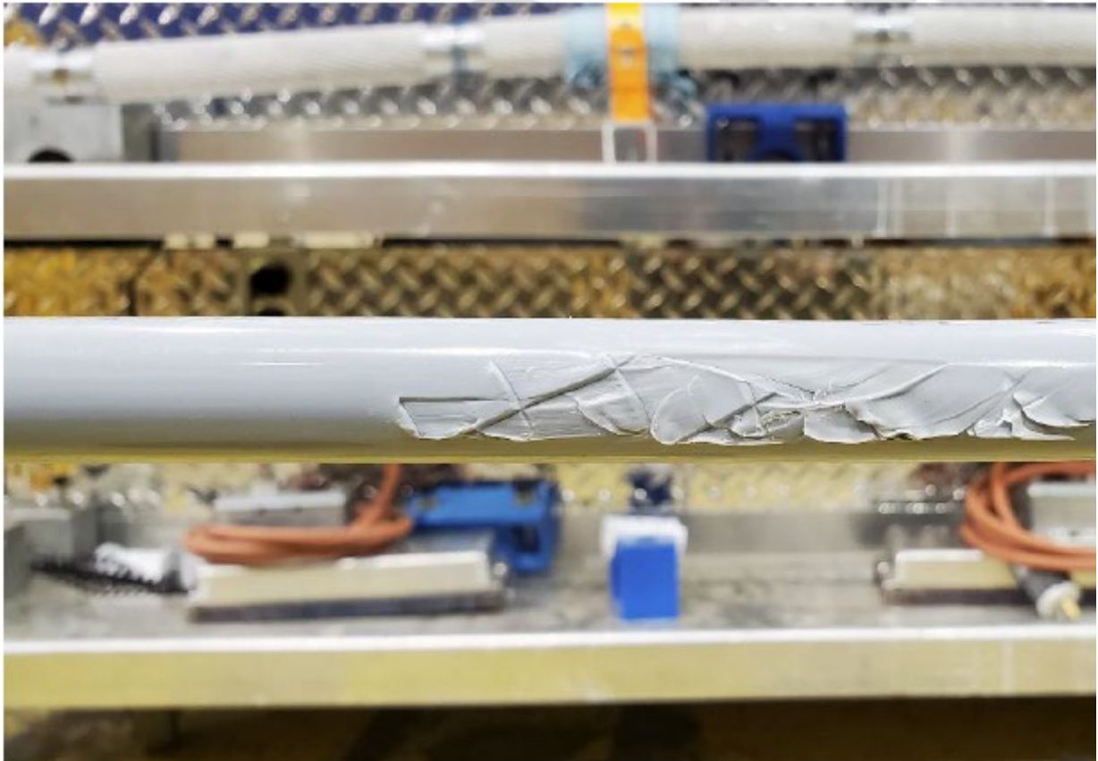
Figure 67. A representative post-test image of a 17-kV ACSR CC showing superficial damage to the polymer sheath caused by slippage.
