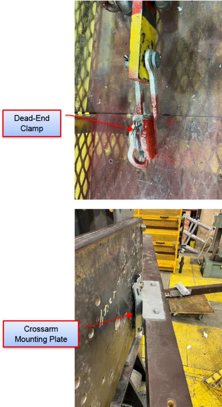
Figure 6-15: Sample 3.2 – Failure Location
