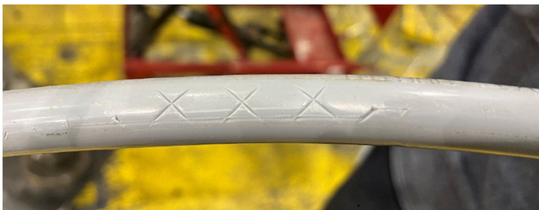
Figure 6-24: Sample 3.4.3 - 15 kV, 1/0 AWG ACSR Condition after Test
