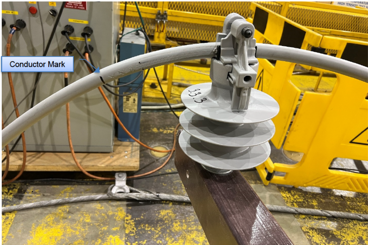
Figure 6-19: Sample 3.3.3 - Insulator and Cross-arm Condition after Test
