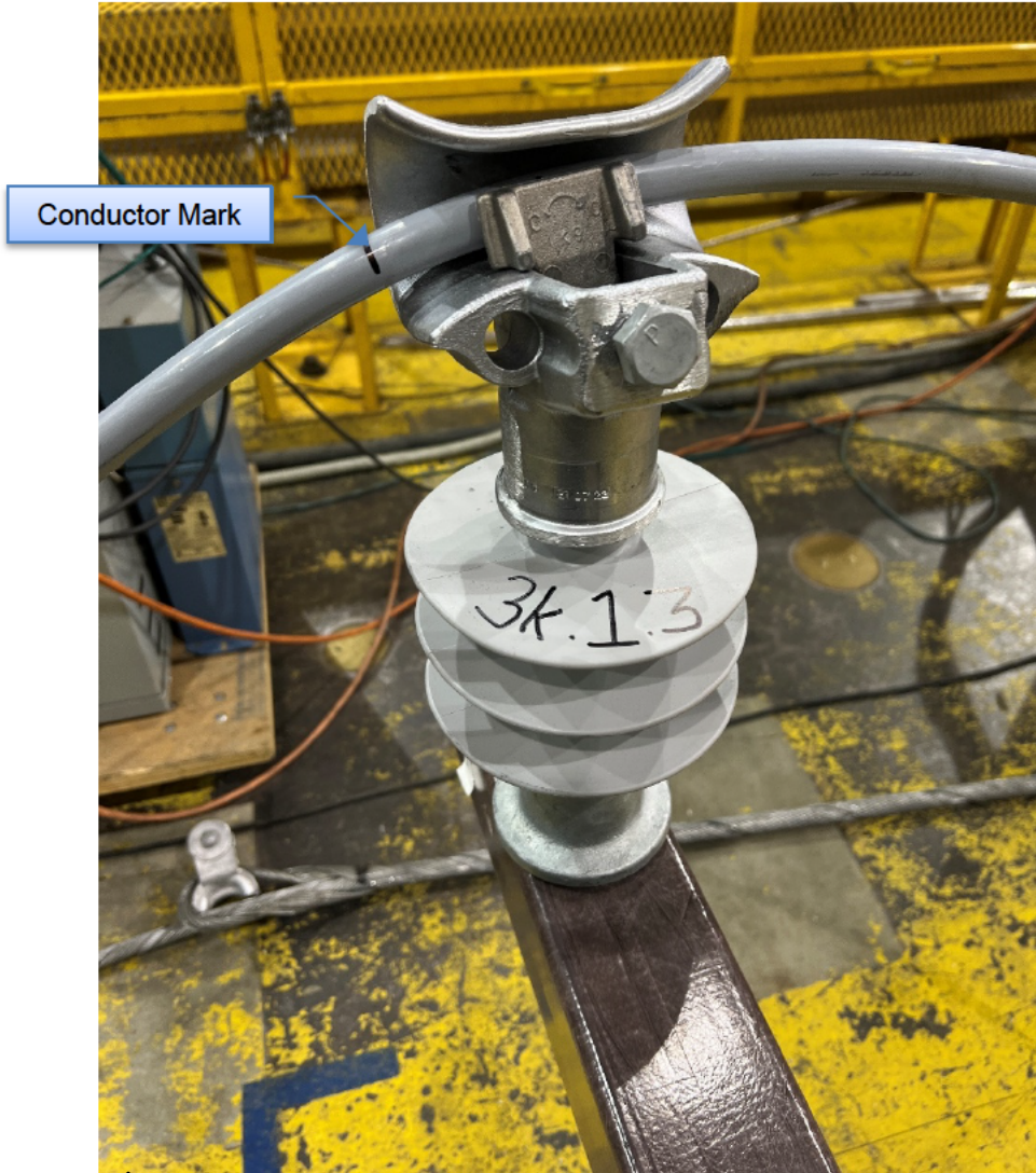
Figure 6-29: Sample 3K.1. – Insulator and Cross-arm Condition after Test
