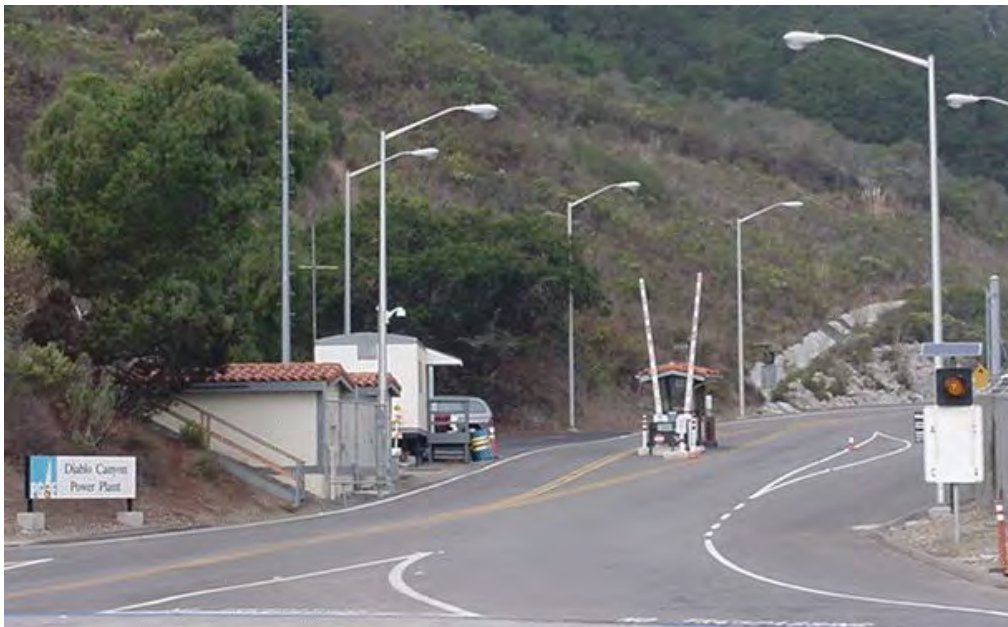
Figure 4-77: Avila Gate Guard House
