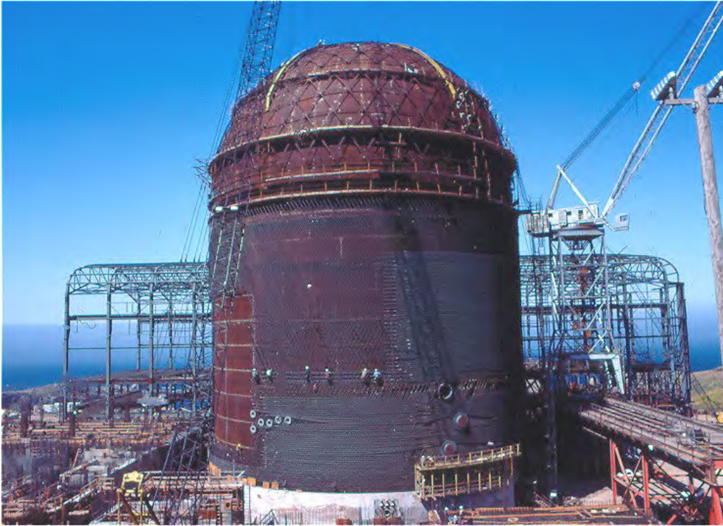
Figure 4-56: Unit 1 Containment, May 1971
