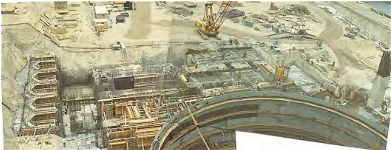
Figure 4-60: Auxiliary Building, May 1970
