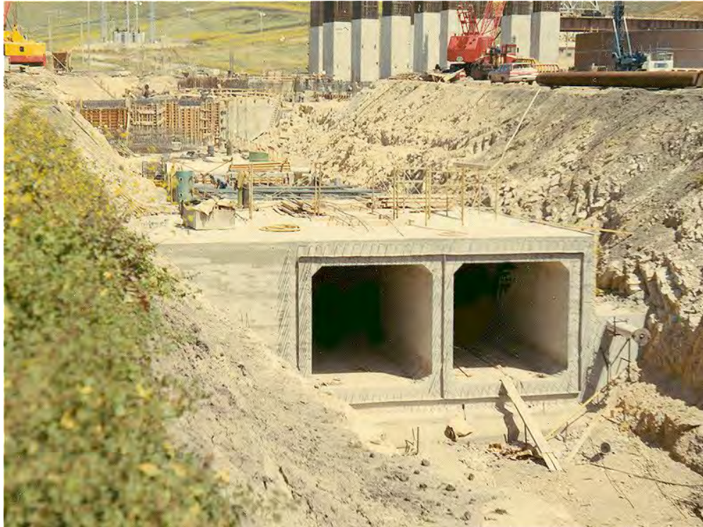
Figure 4-78: Unit 1 Intake Tunnels
