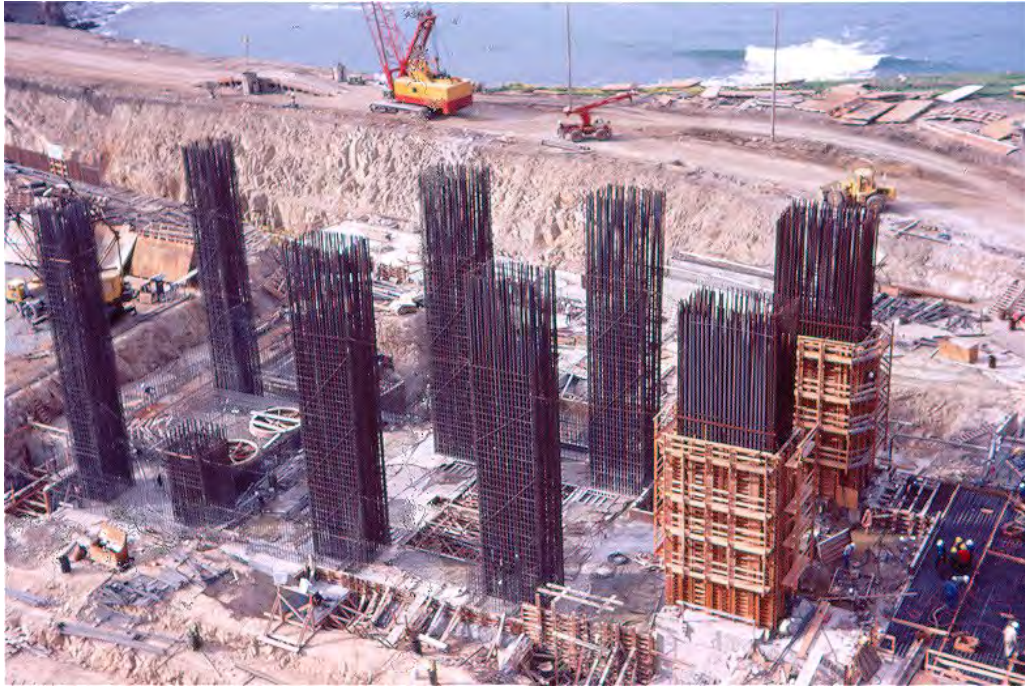
Figure 4-63: Unit 1 Turbine Building, February 1970
