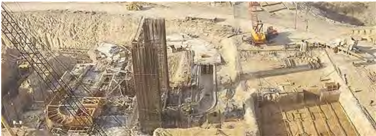
Figure 4-62: Unit 1 Turbine Building, December 1969
