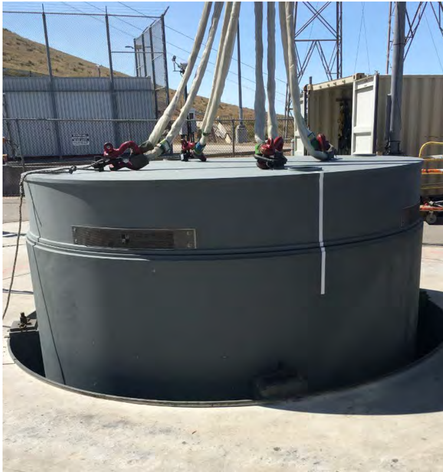
Figure 4-44: Cask Transfer Facility (CTF)
