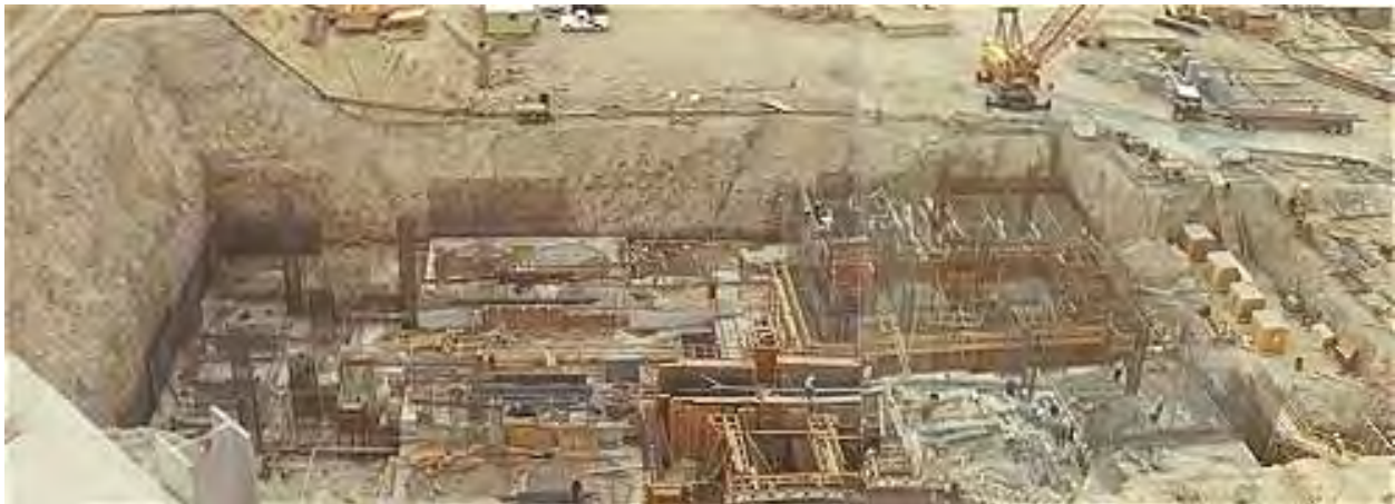
Figure 4-58: Auxiliary Building, January 1970
