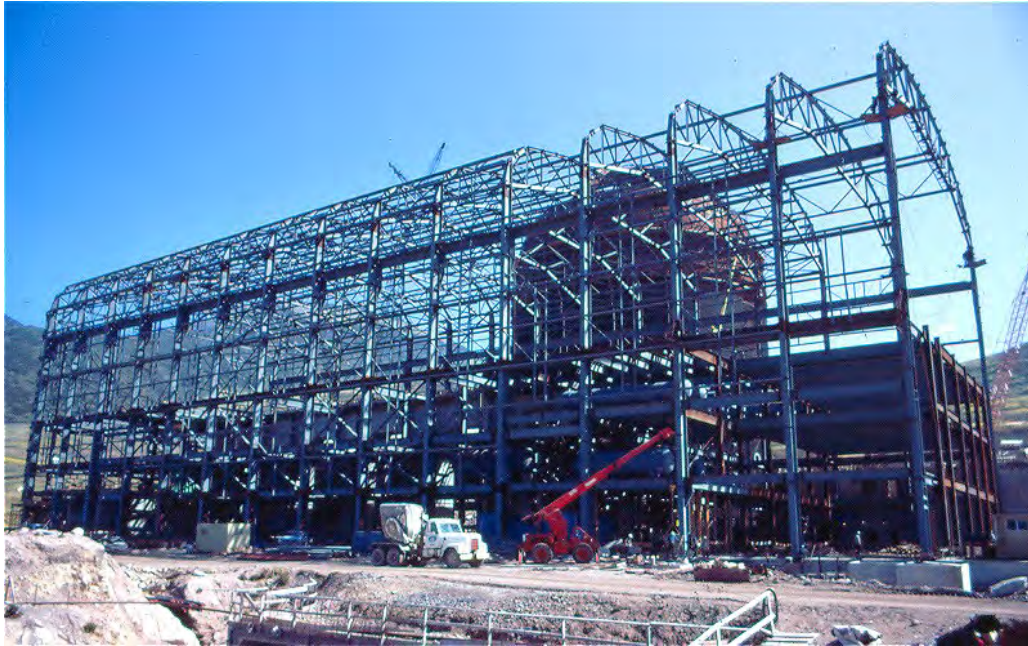
Figure 4-65: Unit 1 Turbine Building, April 1971
