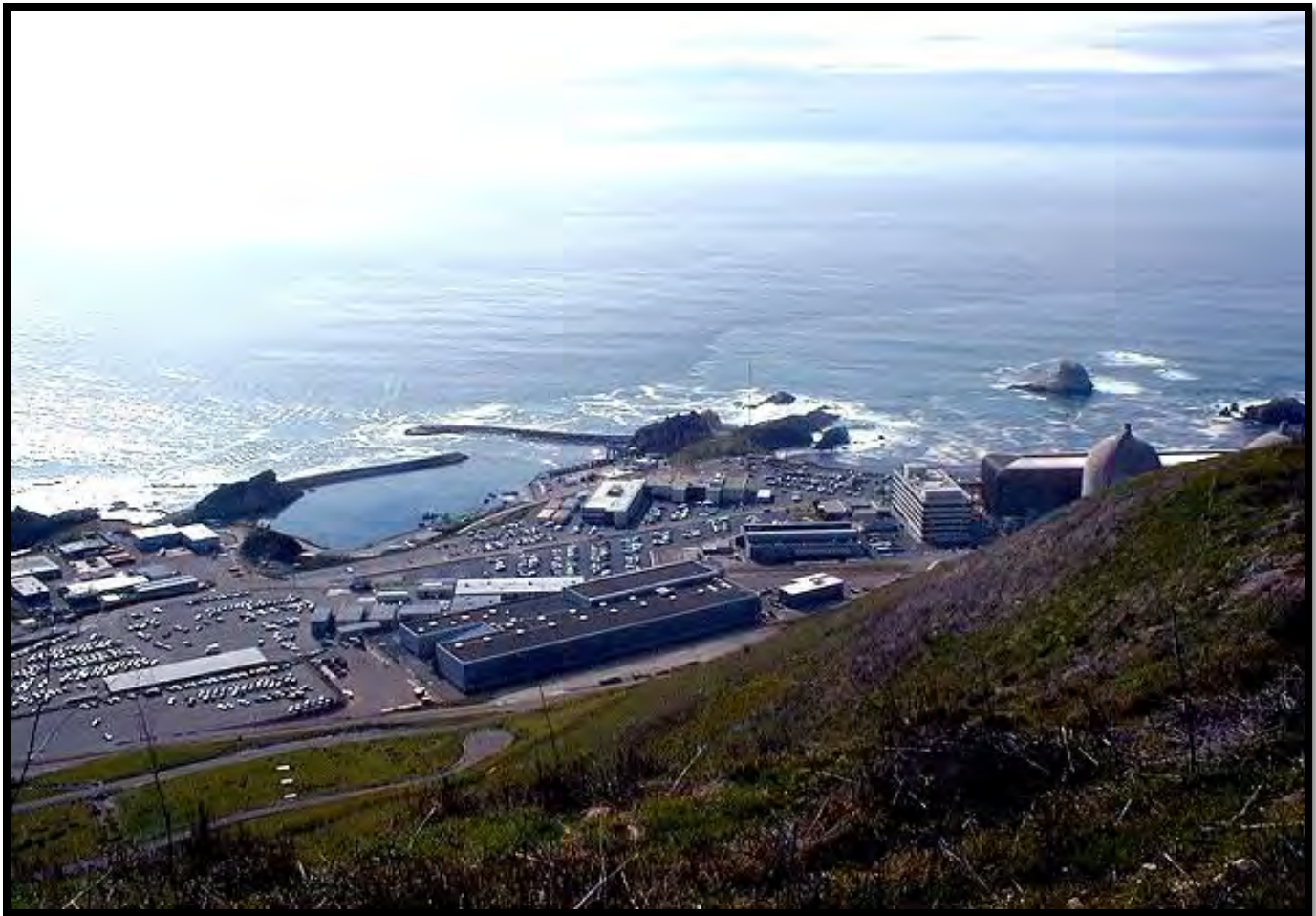
Looking west at the DCP site. The prominent building in the foreground is DCP's Warehouse.
