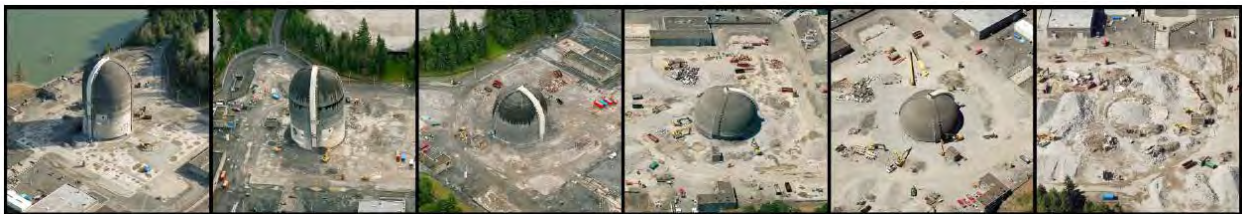
Figure 4-57: Trojan Nuclear Power Plant Containment Shell Demolition
