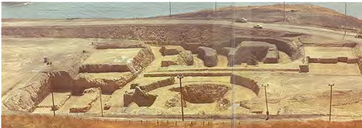
Figure 4-53: Unit 1 Power Block Initial Excavation, June 1969
