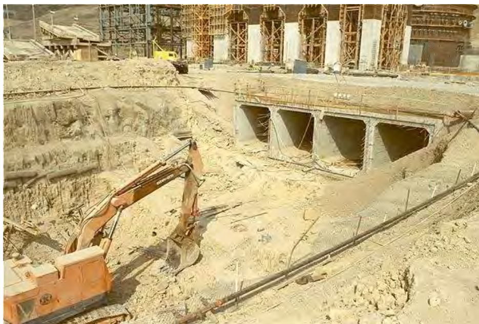
Figure 4-79: Unit 1 and 2 Discharge Tunnels
