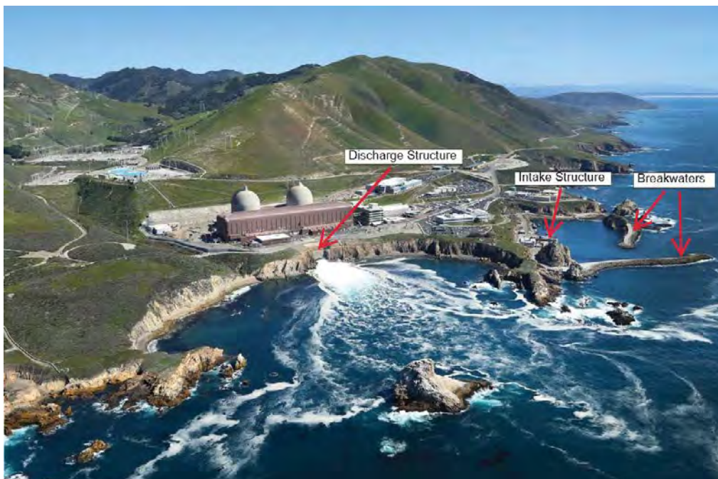
Figure 3-6: DCCP's Intake Structure, Breakwaters, and Discharge Structure Looking Southeast
