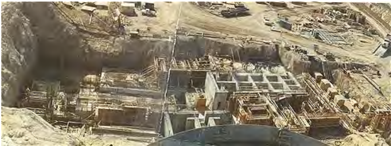
Figure 4-59: Auxiliary Building, March 1970
