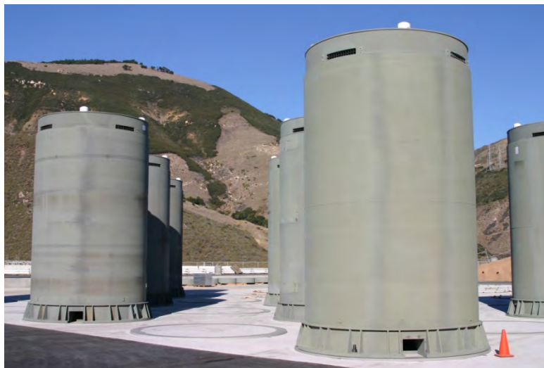
Figure 4-41: Storage Over-pack Dry Casks Containing Spent Fuel Stored at ISFSI (HI-STORM)
