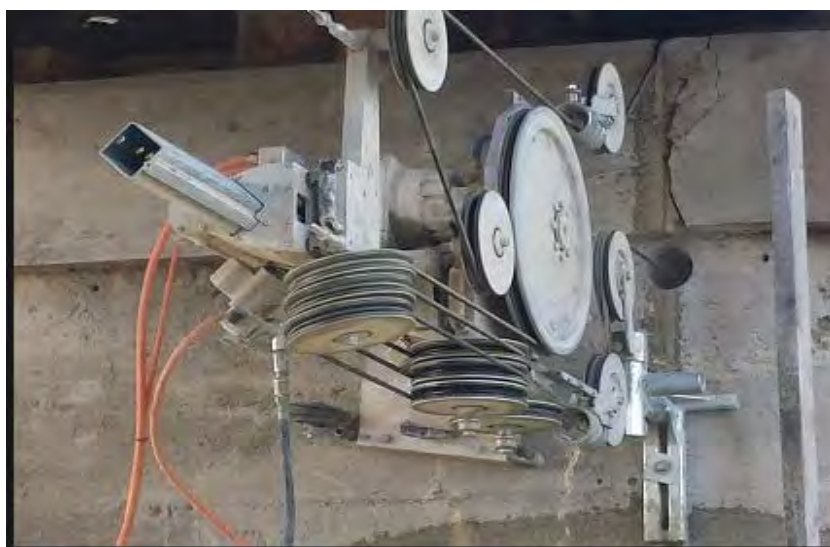
Abrasive wire saw equipment setup to cut small concrete sections
