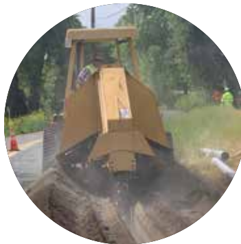
Alvah Group, Inc.: Undergrounding Fire Hardening
