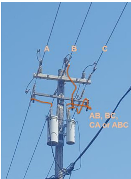
Figure 2: Phasing Options on a 3-Wire Circuit
