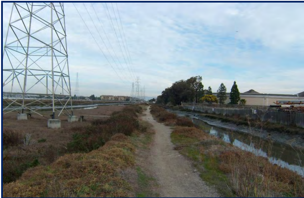
Subject proposed easement area facing east, generally in the middle of the proposed easement
