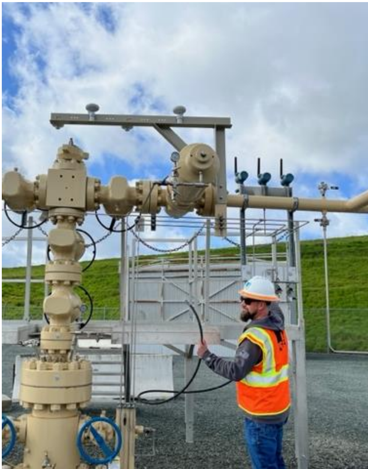
Figure 4: The near field fixed monitoring project is testing the technical specifications and leak detection capabilities of various methane sensors for continuous monitoring of wellheads at underground storage facilities. Incorporating fixed methane monitors can reduce operating risks though early detection of high-risk methane leaks, potentially preventing loss of containment.
