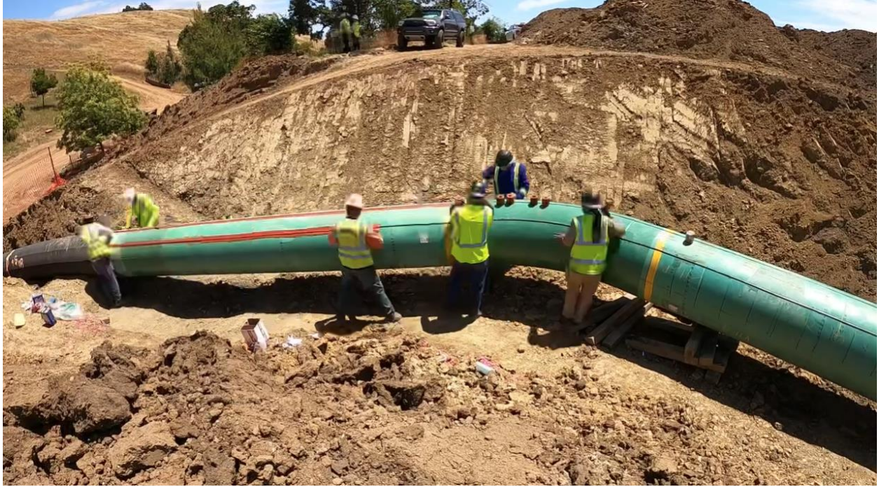
Figure 3: Funded by a US Department of Transportation/PHMSA University grant and Small Business Innovation Research funds, the project involved the first of its kind installation of a distributed fiber optic sensor monitoring system to assess pipeline strain associated ground movement at the Calaveras fault-crossing south of San Jose. The image captures the installation of the fiber optic sensor on the pipeline.
