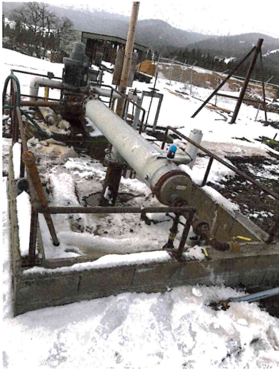
Figure 1. Strainer Assembly at Upper Pond
