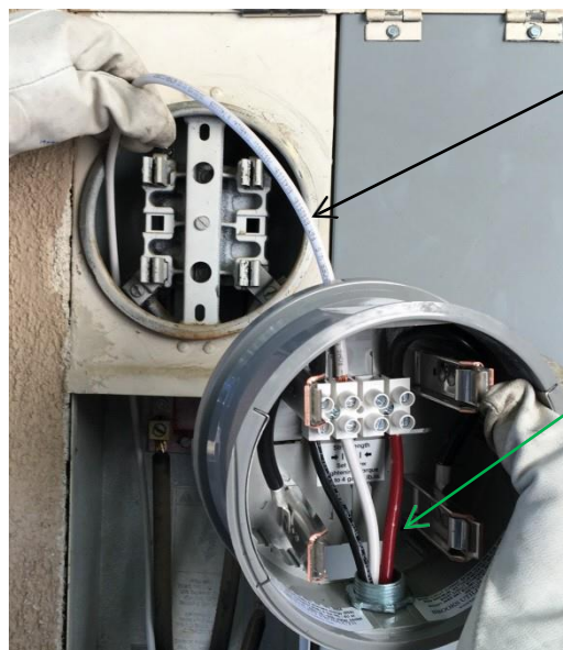
Figure 5. Extend Insulated Wires Past the LFNC Conduit
