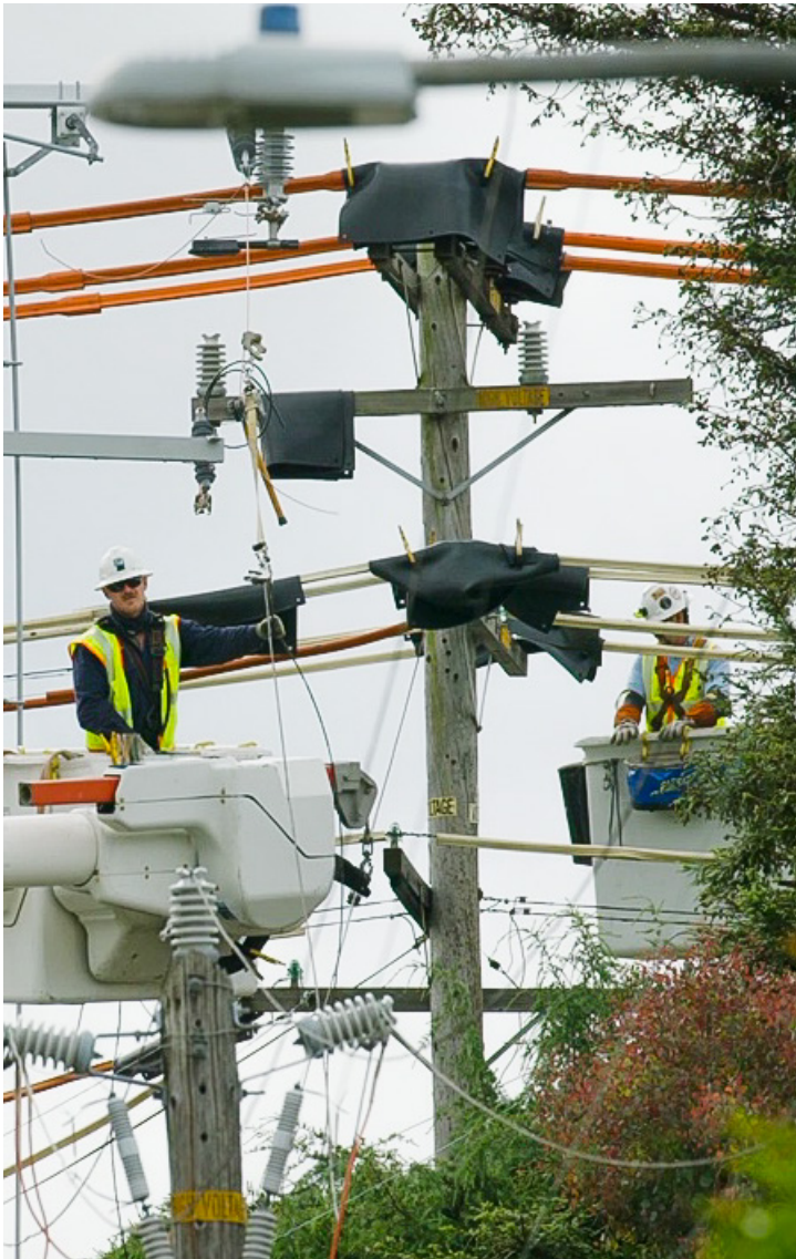
PG&E crews in the field
