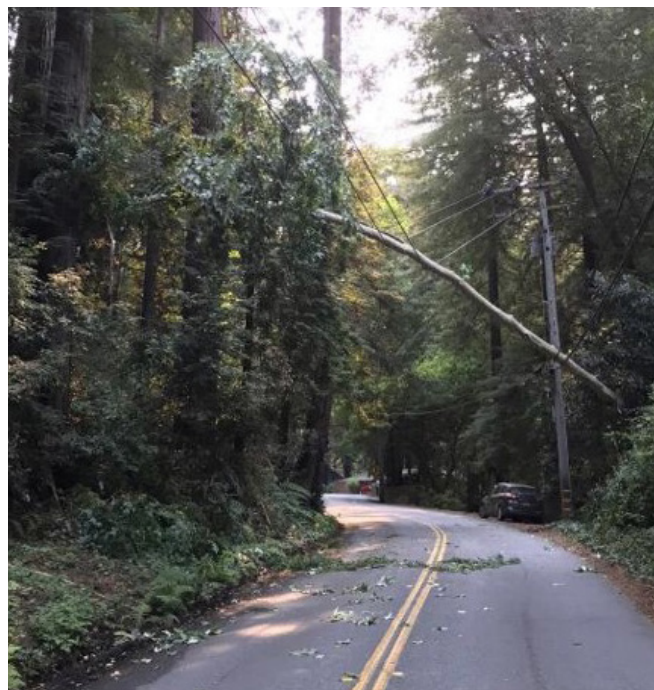
Example of a vegetation hazard that resulted in an EPSS outage last month
