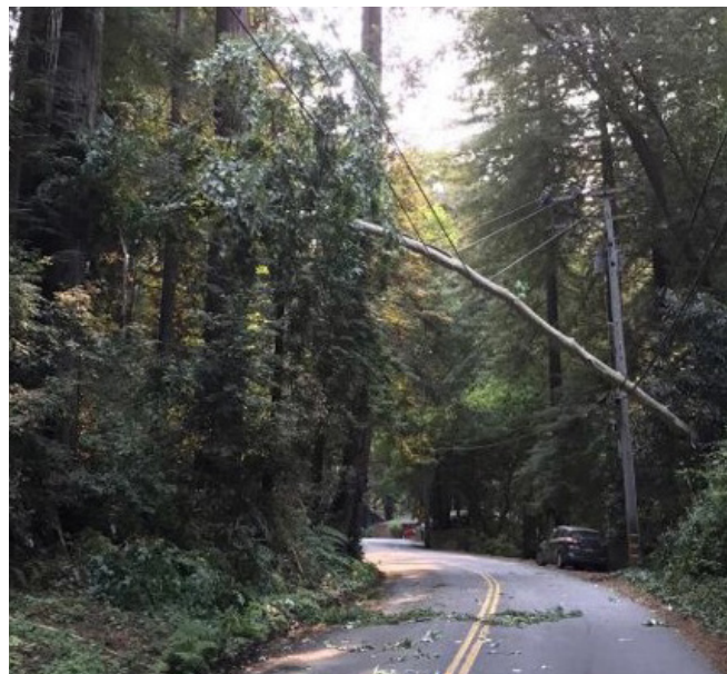
Example of vegetation hazard that resulted in an EPSS outage last month
