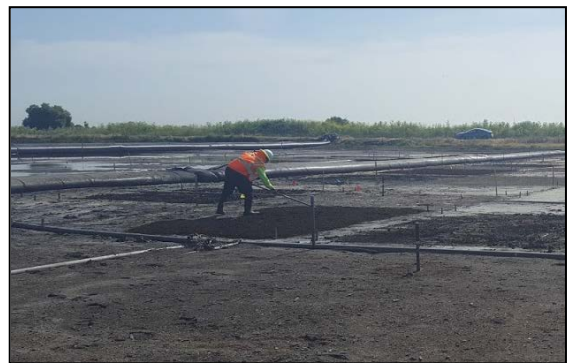
Workers reseeded area to promote plant growth and overall health. They will also use a rototiller on a portion of the study to see if that would improve plant health and break down of the waste.
