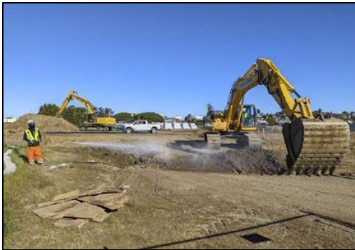
Crews excavating contaminated soil while spraying water to control dust.
