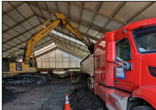
Excavated soil is loaded onto a truck for off-site disposal.
