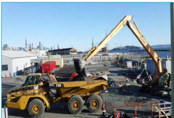
Soil removed during ISS preparatory work is transferred to the on-site stockpile area
