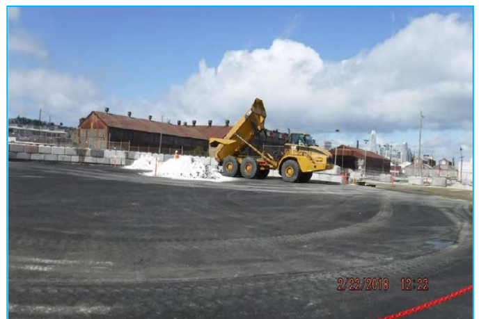
Soil removed during ISS preparatory work is transferred to the on-site stockpile area
