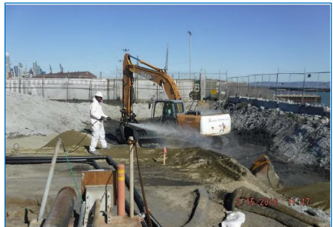
Crew member performs dust and odor control misting
