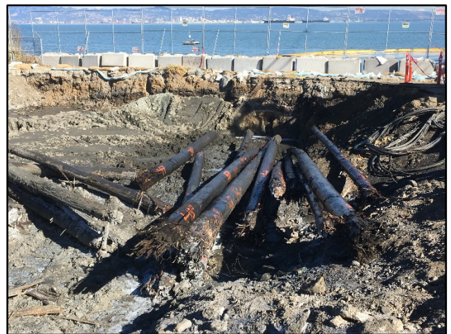
Removed wood piles
