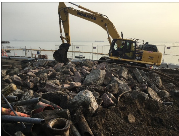
Breaking down concrete for transport and disposal
