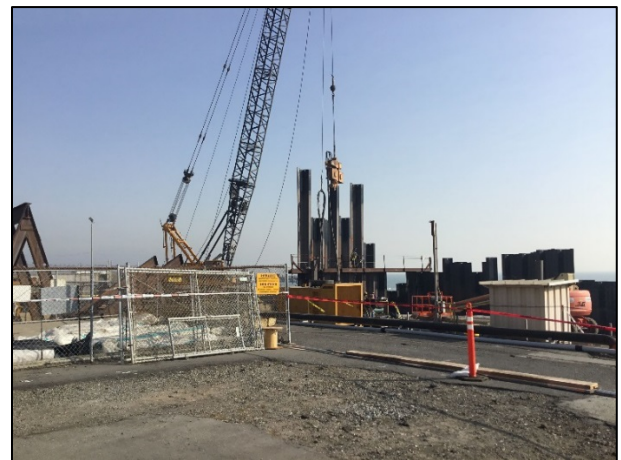
Installing steel sheeting along the shoreline
