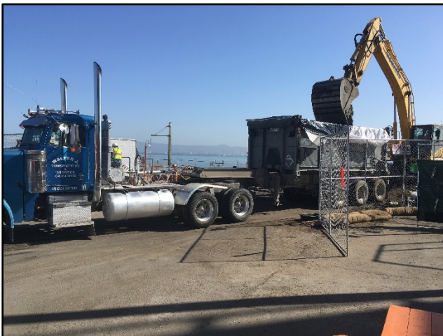
Loading debris and soil for transport and disposal
