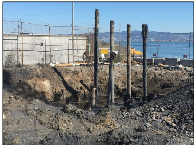
Removing wood piles, such as those shown above
