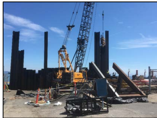
Installation of steel sheeting along the shoreline
