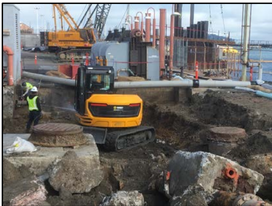
Removal of underground utility lines
