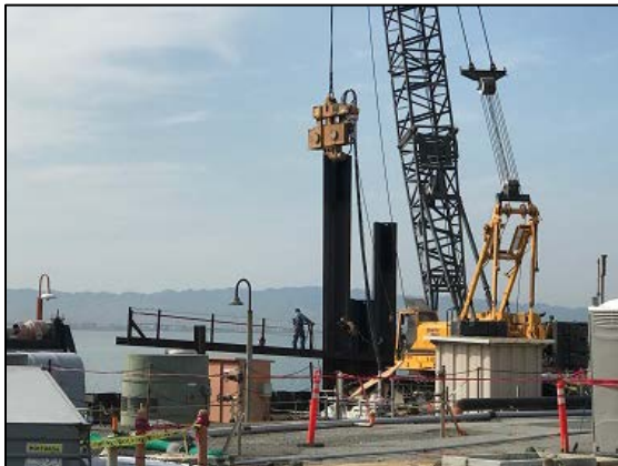
Installation of steel sheeting along the shoreline
