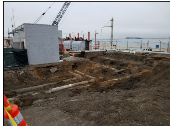
Exposed underground utility lines for removal or replacement
