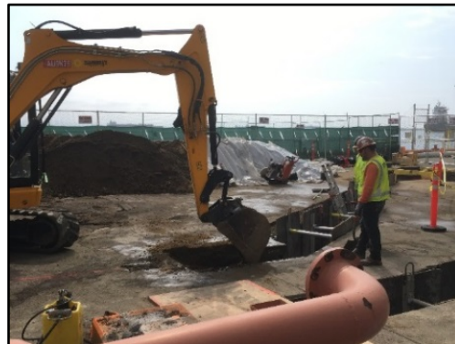
Removing underground utility lines
