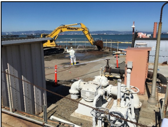
Soil Excavation in Preparation for Installing Steel Sheet Piles
