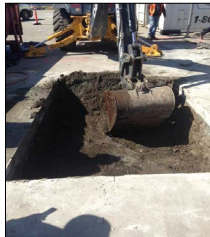
Workers will dig small pits to observe conditions underground.
