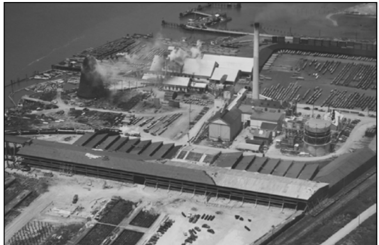
The former Eureka manufactured gas plant in June 1948.
