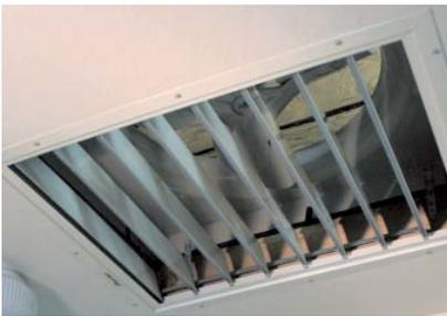
Typically, Whole House Fans are installed in a hallway ceiling (over the top of the ceiling joist) in a horizontal position to expel hot air from the house into the attic and out the attic vents. If the configuration of the house does
