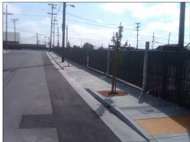
West Front Street after remediation – August 2010
