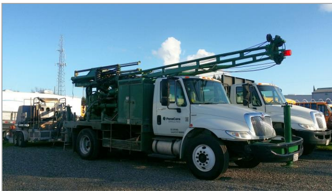
A drill rig (left) will be used to install new wells.
