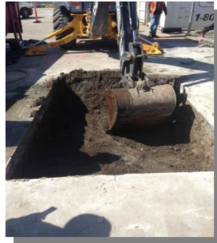
Trenching will provide information on subsurface conditions
