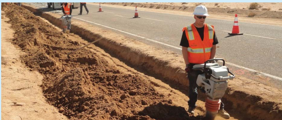
PG&E crews install new pipeline to provide freshwater to Hinkley School.
