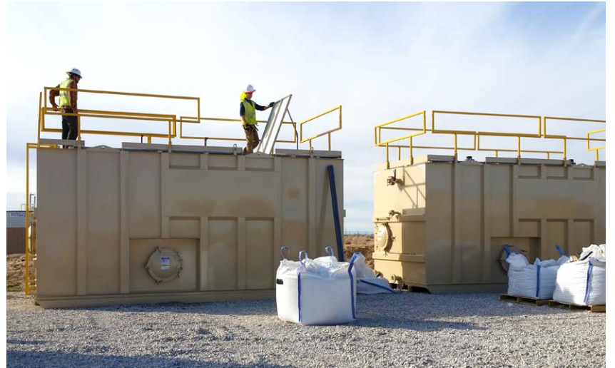
Workers prepare the 10,500 gallon tanks for pilot testing.
