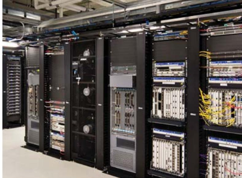
Energy-intensive server labs feature many energy conservation measures. Here in-row, water-chilled fan coils and overhead supply air ducts minimize the mixing of hot and cold air to reduce the lab's overall cooling load.
