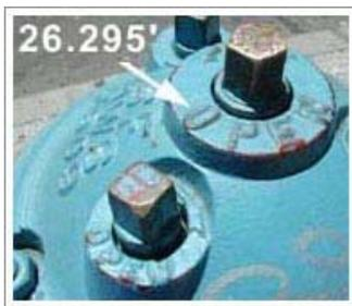
Figure 3: Detail of reference point location (*Benchmark 1*)
