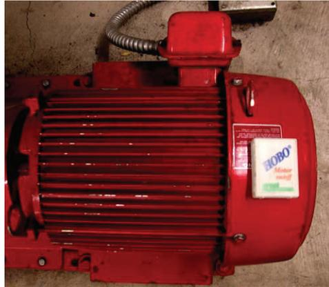
Figure 4: Motor logger installed on pump motor
