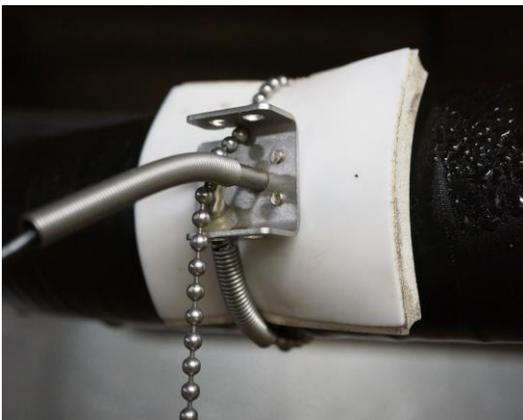
**Figure 9b** (Optional) Properly mounted RTD sensor with insulating pad and chain clamp
