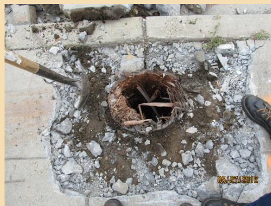
After extraction showing below ground deterioration
