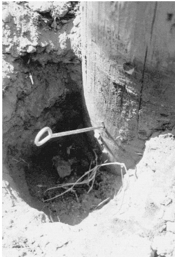
Figure 3. Using a Shell Thickness Gauge
