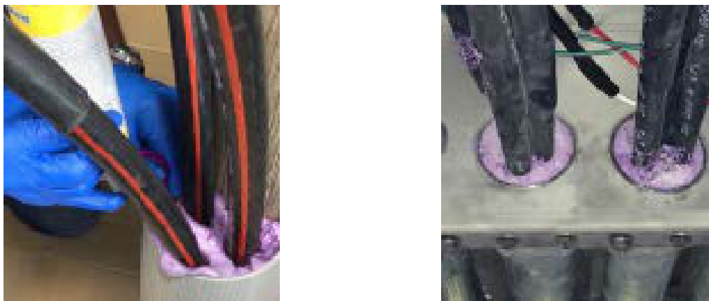
Figure 46 Example of Polywater ® AFT Installation in Riser Poles and Raceway Entrances
