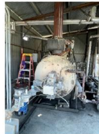
Boiler-burner for NG-H2 blending
