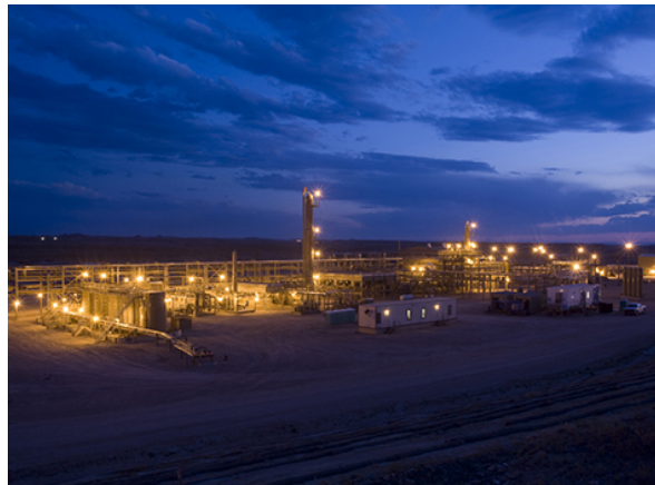
Figure 1 UOP Russell modular cryogenic plant
