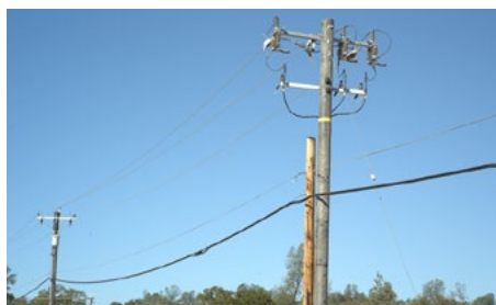
Installing more poles to support the weight of covered powerlines
