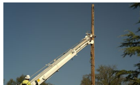
Removing poles and overhead lines that are no longer needed
