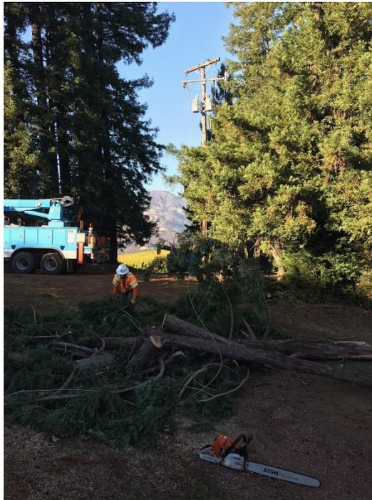
*Figure 2. Near Calistoga, Sonoma County. Primary conductor damaged by fallen tree limb.*
