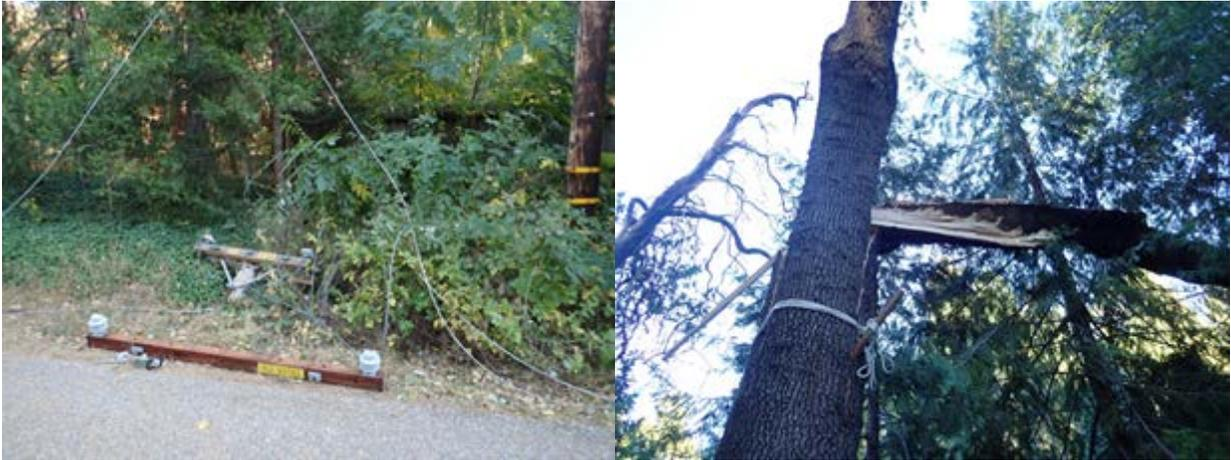
*Figure 1. Foresthill, Placer County. Pole, cross-arm and conductor damaged by split tree.*
