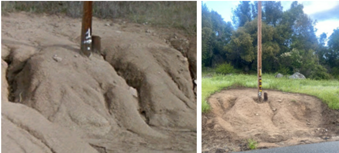
Figure 3. Signs of Severe Erosion
