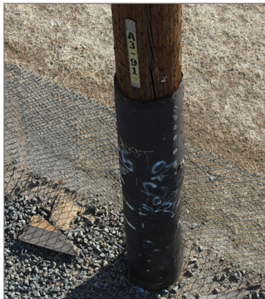
Figure 16. Fiber-Wrapped Wood Pole
