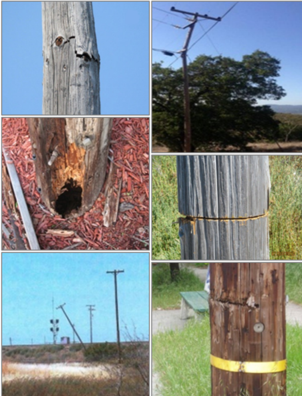
Figure 18. Examples of Visual Inspections Requiring Escalation
