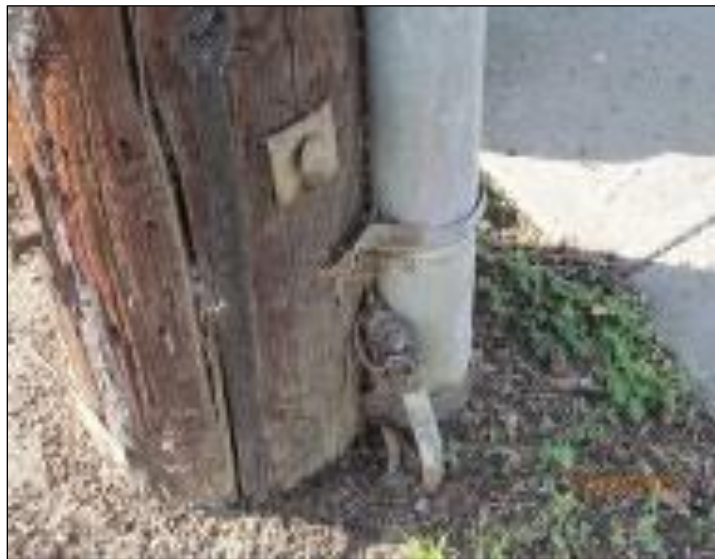
Figure 14. Example of OH Inspection Minor Work
