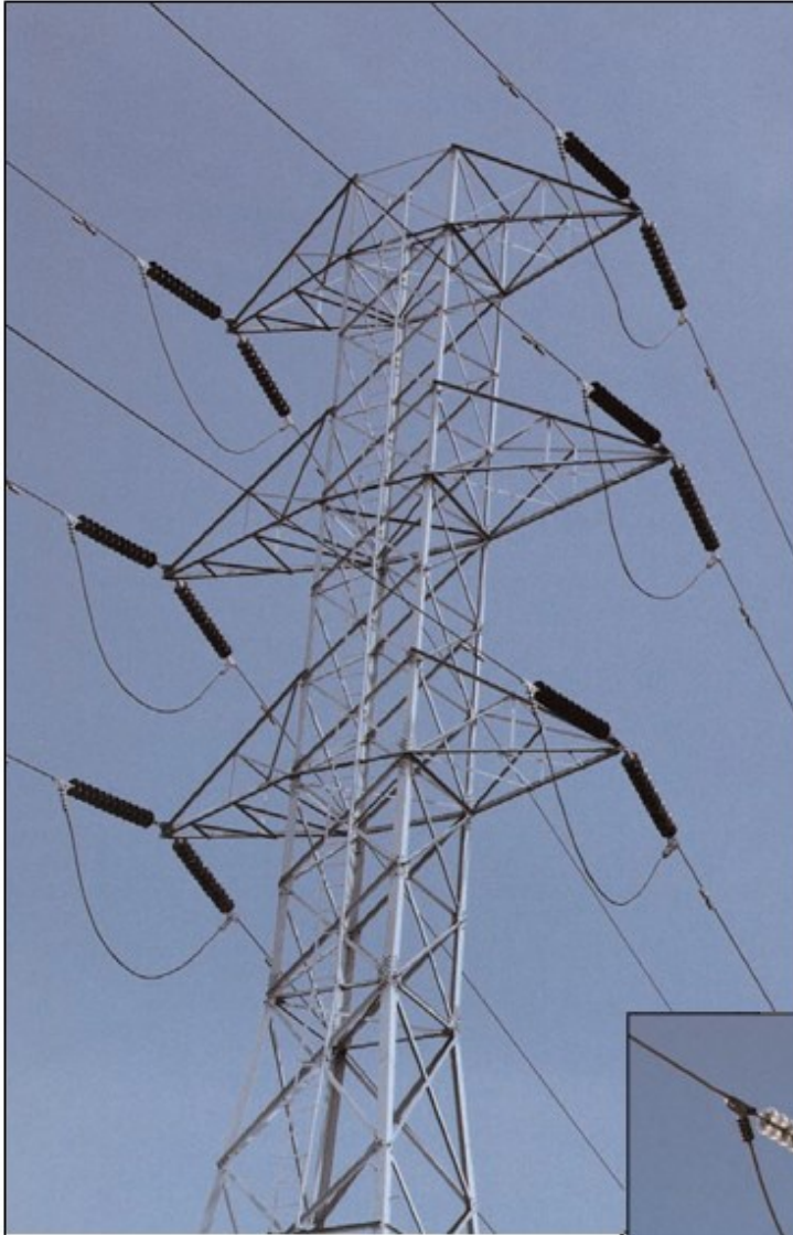
Figure PLC-34: Dead-end Tower
