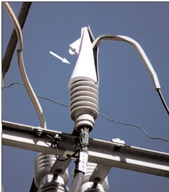
Figure PLC-23: Close up of Squirrel Guard
