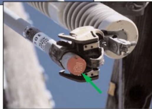
Figure B-17: SMU-20 - Fuse Detail
