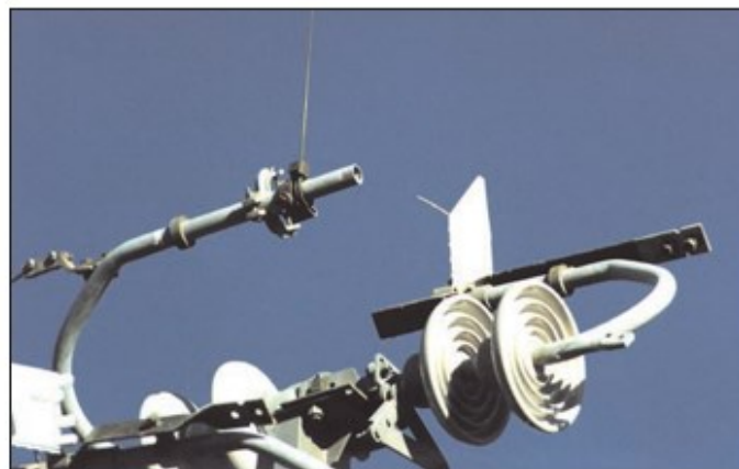
Figure B-23: 600 Amp KPF Air Switch, Triangular Construction (Open Position)
