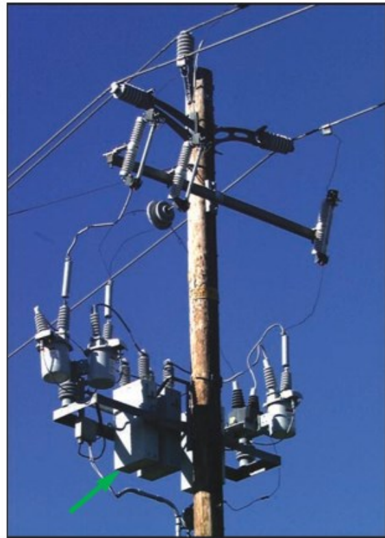
Figure B-51: Capacitor Unit
