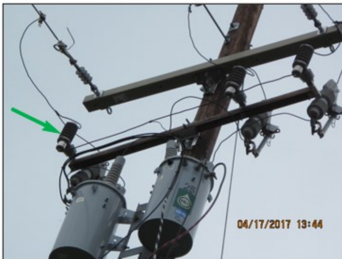
Figure B-87: Siemens Lightning Arrester
