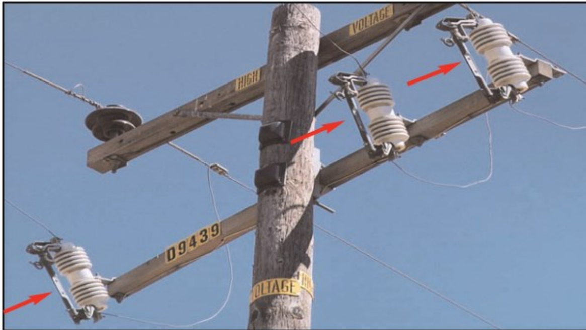
Figure NE-11: Arm Mounted Cutout with Solid Blade Disconnect (closed position)
