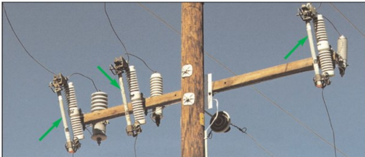
Figure B-18: Arm Mounted Cutout with SMU-20 Fuses
