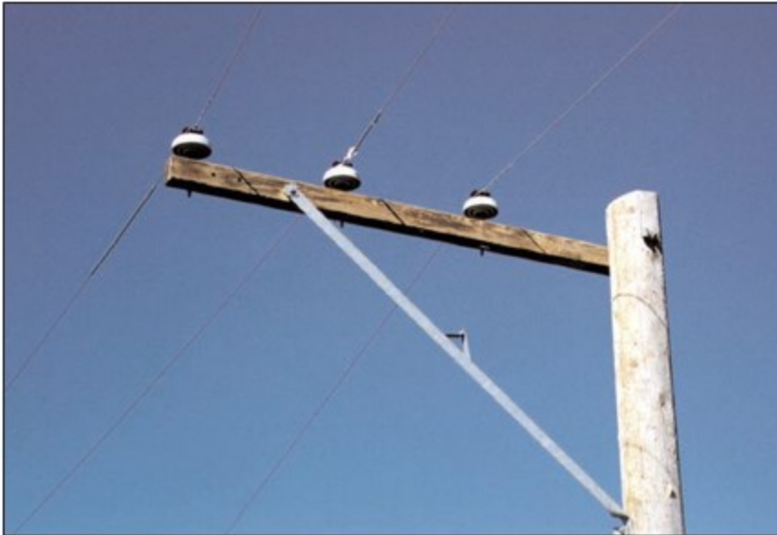
Figure PLC-3: Alley Arm
