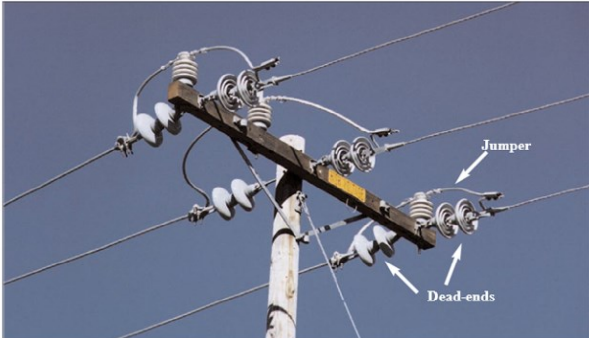
Figure PLC-7: Crossarm Double Dead-end
