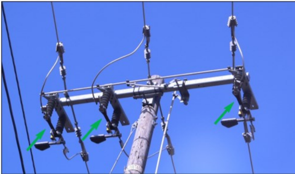
Figure B-40: 27kV Inertia Line-Boss Underarm Side Break Switch (Closed Position)
