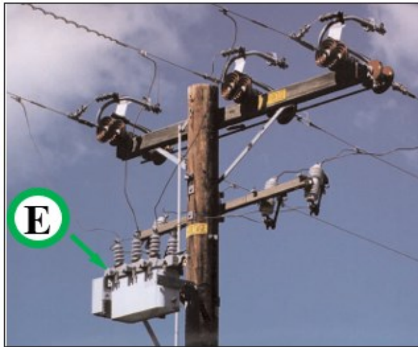
Figure B-45: Sectionalizer with Solid Blade Disconnects
