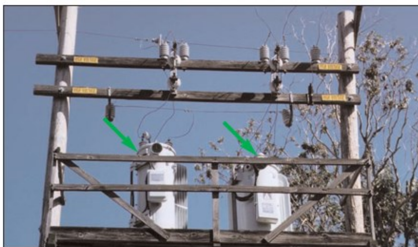
Figure B-49: Voltage Regulator
