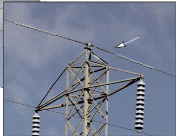
Figure PLC-37: Close-up of Static Line
