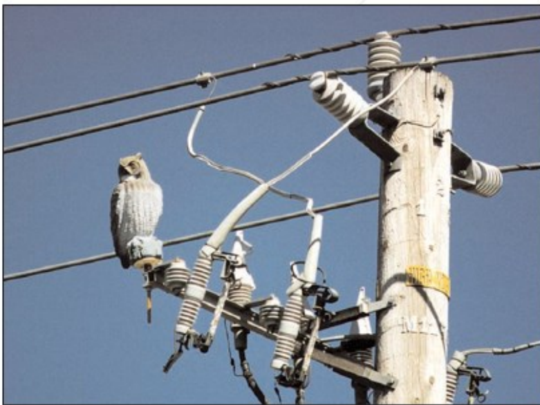
Figure PLC-20: Anti-Perch Owl
