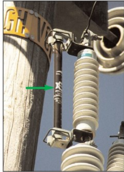
Figure B-11: Liquid Filled Fuse
