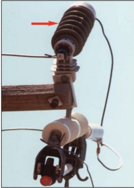
Figure NE-23: Non-Porcelain Lightning Arrester
