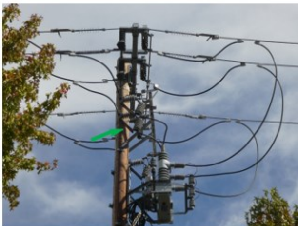
Figure B-47: 600A Disconnect. It is non-exempt equipment as part of recloser installation
