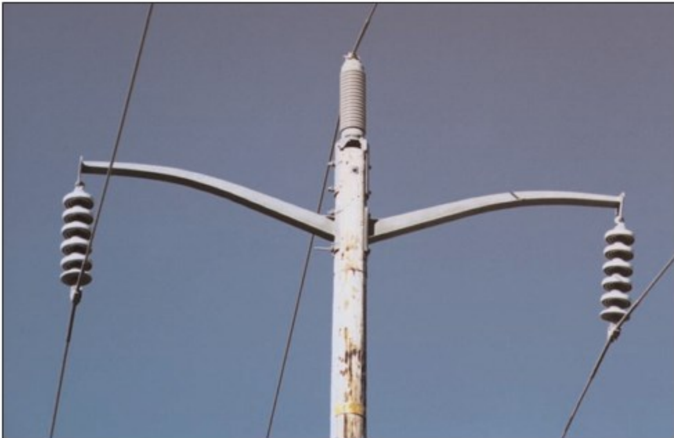
Figure PLC-31: Gull Wing
