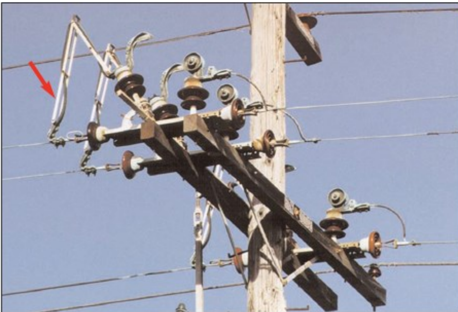
Figure NE-39: Grasshopper Air Switch (open position)
