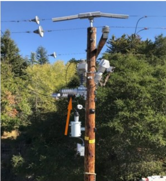
Figure A-2: Fusesaver with in-line solid blades Arm Mounted Cutout
