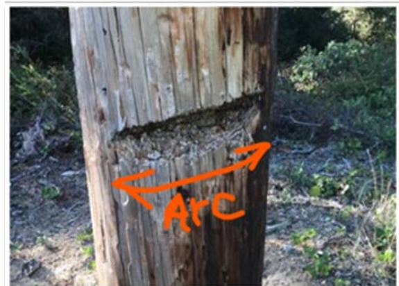
Figure 2: Definition of Crosscut Arc Length
