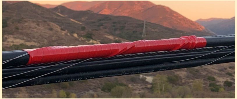
After - Snip Lashing and Tape
