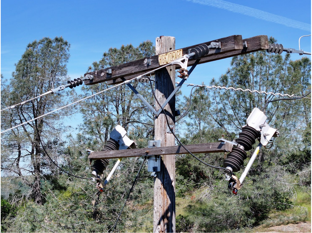
Figure 8 Incident Location #1 - Pole #1 with new fuses. Photo taken by Ignition Investigator on April 22, 2024.
