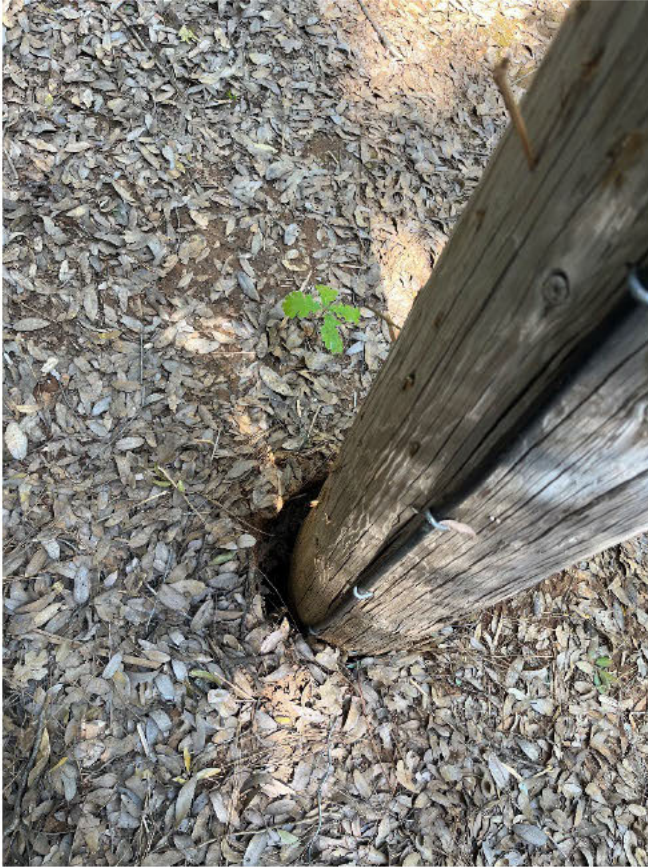
Figure 4 Base of Pole #3 showing the gap created from the forceful movement of the pole when the dozer snagged the guy wire. Photo taken by ignition investigator on April 22, 2024.
