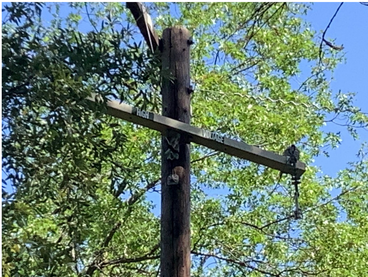
Figure 6 Pole #2 (SAP Pole ID 103320076) - Incident Location #2. Crossarm was damaged when guy wire had been contacted by the dozer, the force pulling the conductor forcibly before it failed. Photo taken by troubleshooter on April 20, 2024.
