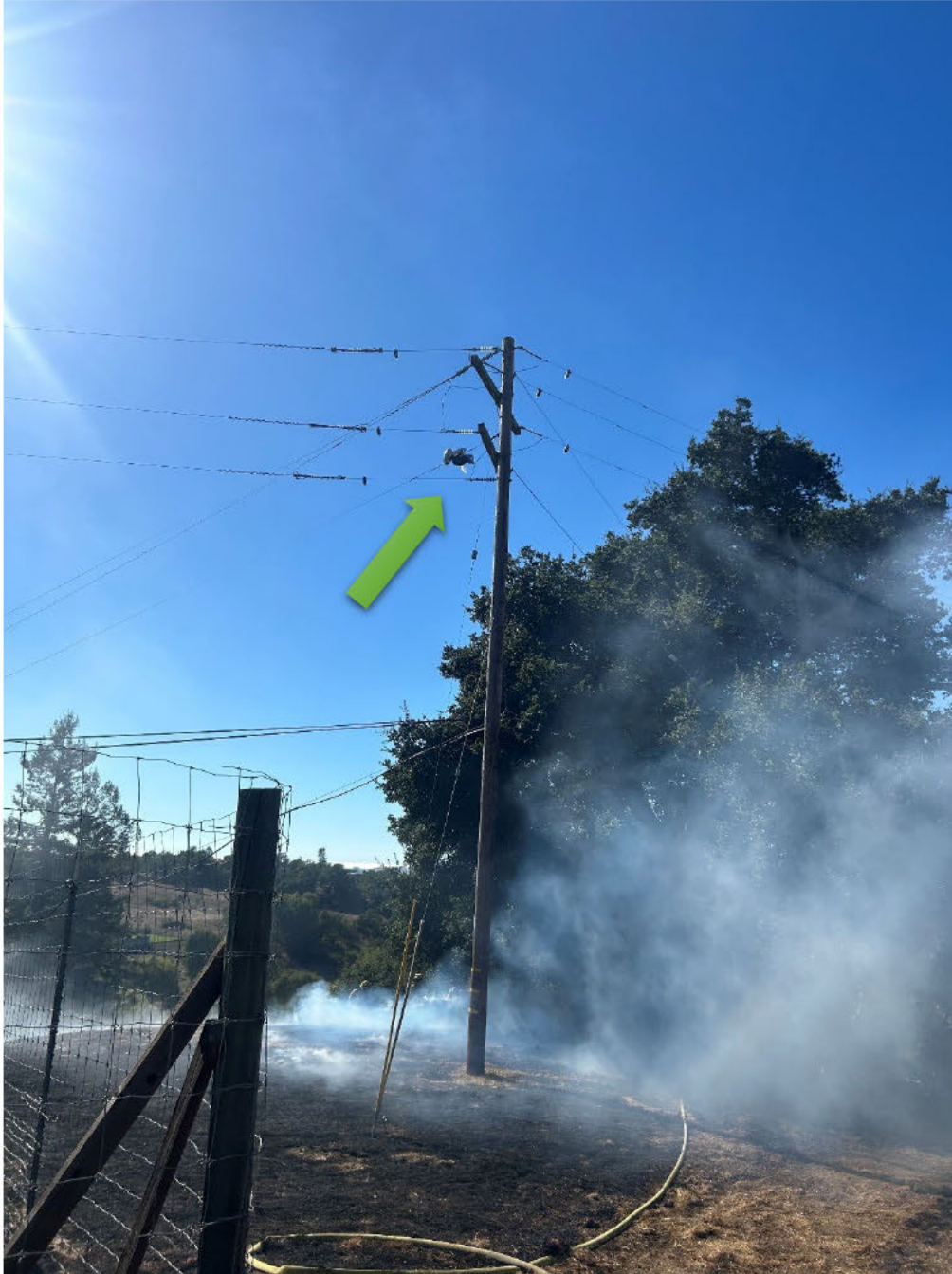
Figure 2 - Photo of the contained fire and burn scar with the balloon contact on the line. Photo taken by troubleshooter on October 142024. SAP Pole ID 103886356
