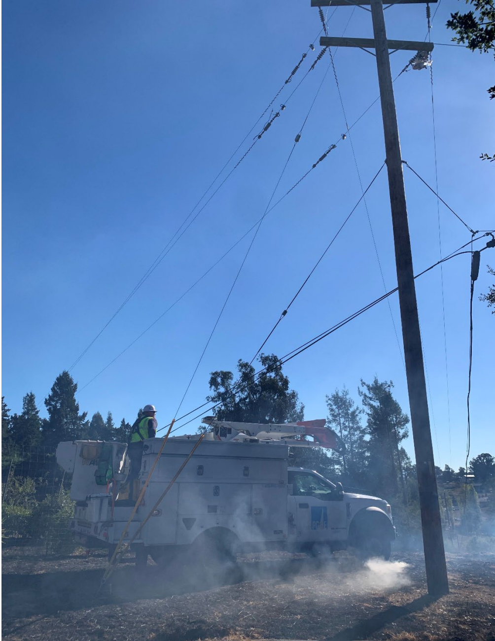
Figure 4- Suppressed fire and PG&E troubleshooter identifying the Mylar balloon prior to removal. Photo provided by troubleshooter on October 14, 2024. SAP Pole ID3103886356
