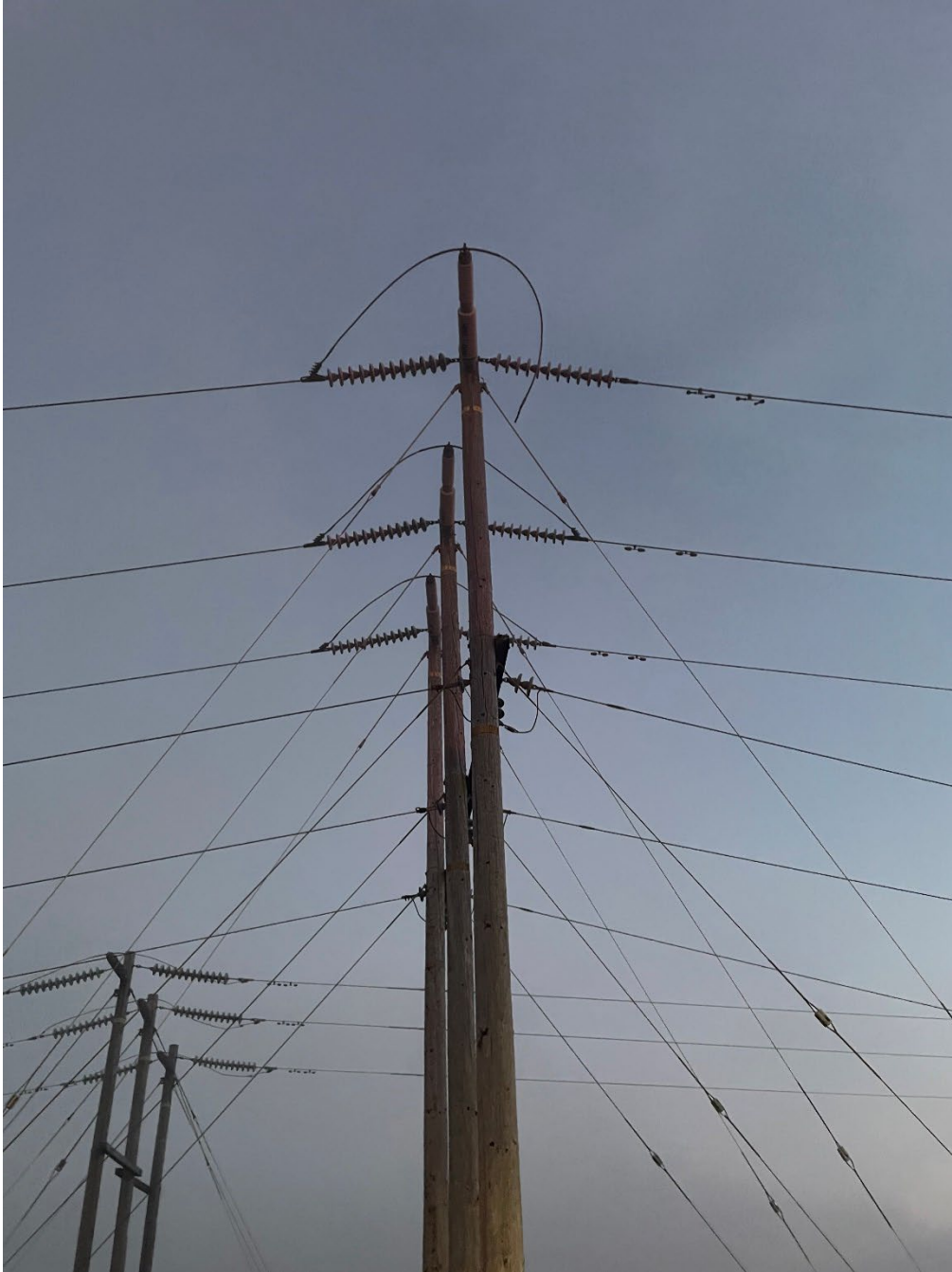
Figure 4 SAP Pole ID 42560786/Structure 004/049 on the Sneath Lane – Pacifica 60kV transmission line, post-ignition. Failed jumper on the southside of pole top. Photo taken by troubleshooter on October 8, 2024.
