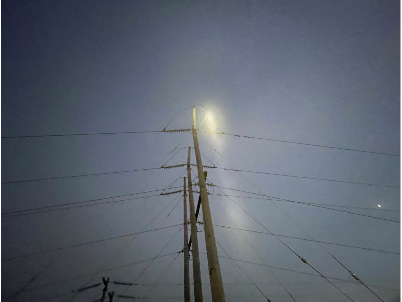
Figure 2 SAP Pole ID 42560786/Structure 004/049 on the Sneath Lane – Pacifica 60kV transmission line. Jumper failure from pole top to south shoe (farthest west phase). Photo taken by troubleshooter on October 8, 2024.
