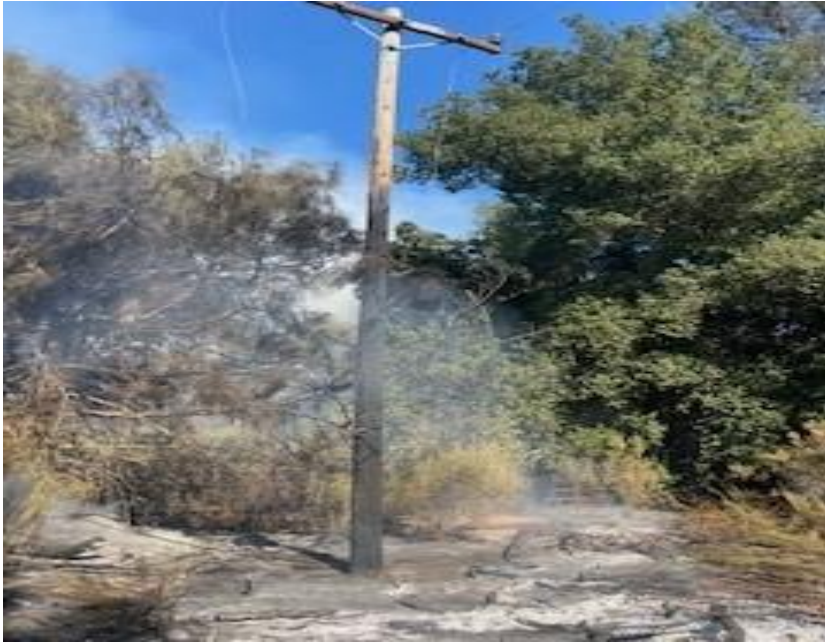
Figure 4 – Brunt and damaged pole SAP pole ID 101690175 (load side). Picture taken by the troubleshooter on September 27, 2024
