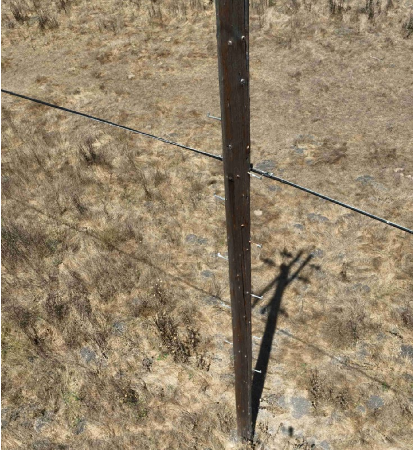
Figure 6 - Photo taken on 08/06/2024 during inspection, showing pole is decayed, base has woodpecker damage
