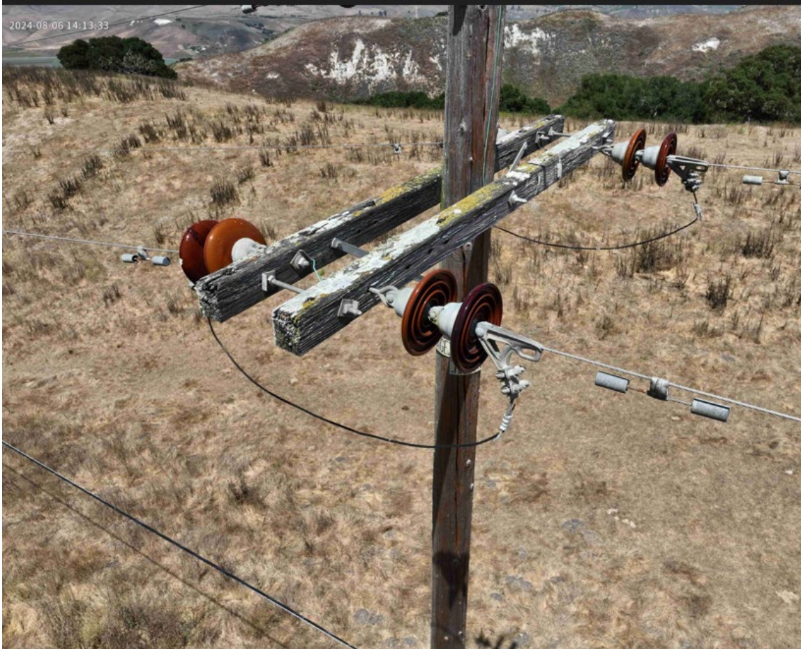
Figure 5 - Photo taken on 08/06/2024 during inspection, showing pole is decayed
